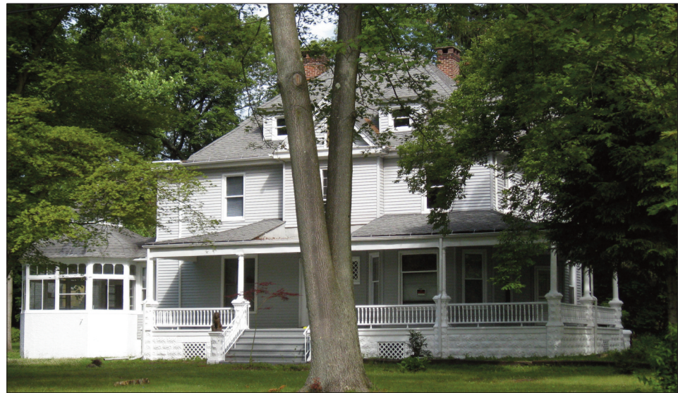
Newly painted, the Maurer Mansion, will be one of Dunellen’s most prominent fixtures in town once fully renovated.
